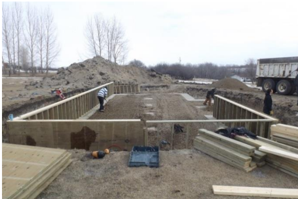
Building foundation one of three new houses for Sioux Valley families
