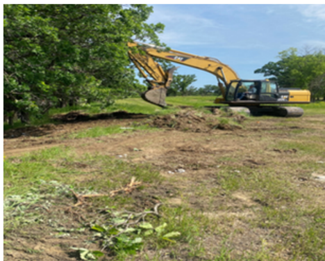
Site cleanup in progress — a backhoe removes large pieces of historic foundation and piles debris along the west edge of the property.
